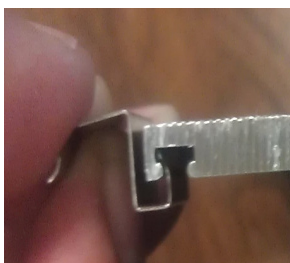
Figure B2: Insert Screen Clip
