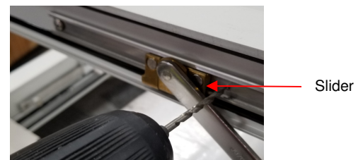
Figure 4: Roto Operator Drill Hole Location (Awning Shown)
