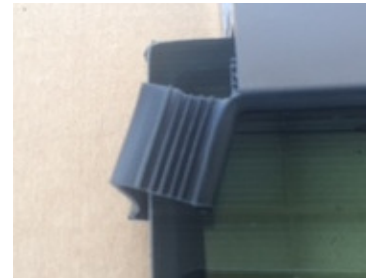
Figure C1: Cut away glazing Vinyl
