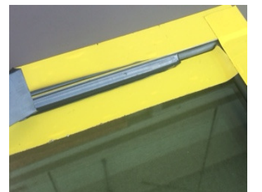
Figure C5: Tool Finish Bead
