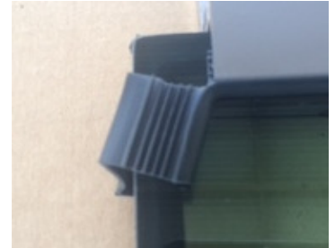
Figure C1: Cut away glazing Vinyl
