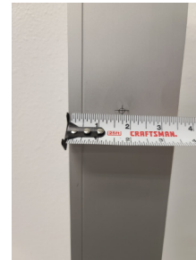
Archetype Narrow Lock Stile with Yoke
