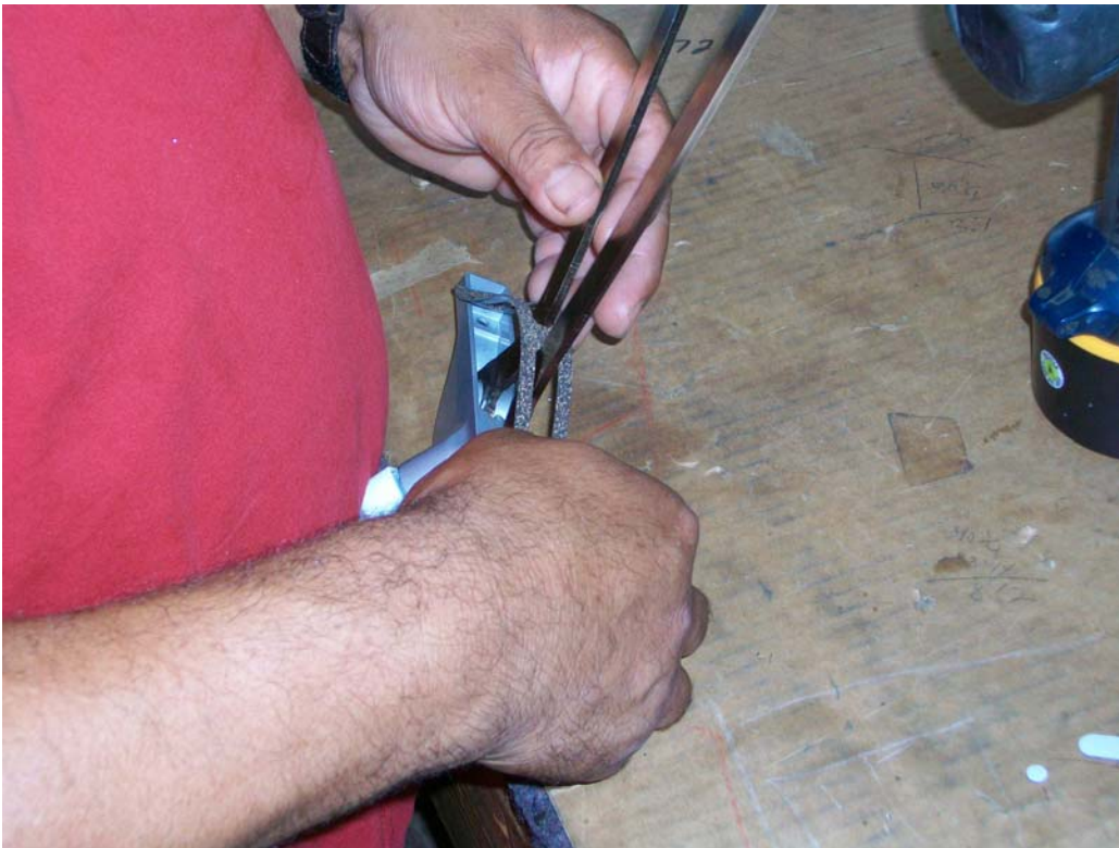
4. Install gasket on pivot shoe
