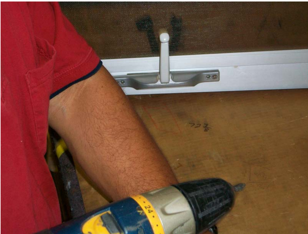
6. Attach pivot shoe with fasteners
