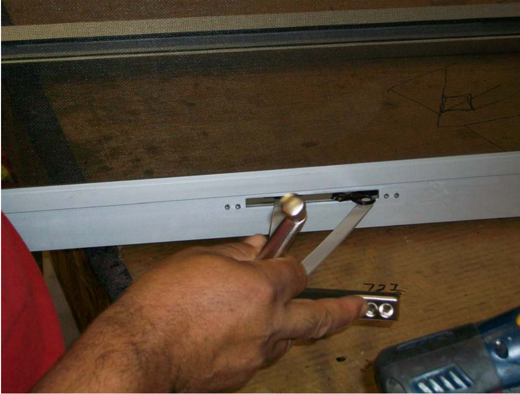
5. Install pivot shoe with SS Arms
